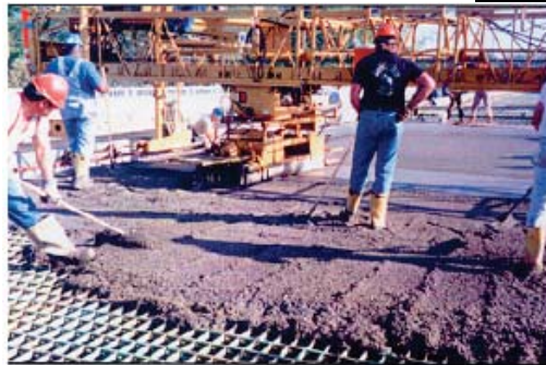
Deck of North Main Street Bridge, Akron, Ohio, received a fusion bonded epoxy coating
